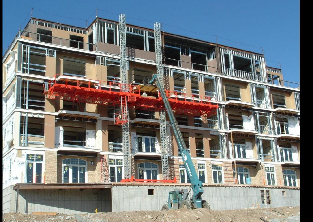
TRANSFERRING MATERIAL FROM **PLATFORM TO BUILDING ONLY** ALLOWED IF THE WORK IS PART OF THE WORK BEING DONE ON THE PLATFORM
